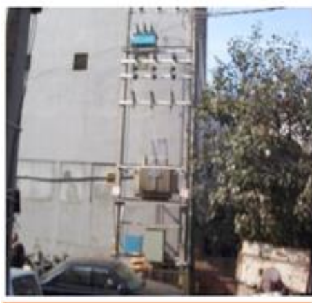
Fig. 1.36 Outdoor Type HT Metering
