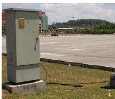
Fig. 1.28 Group Metering-Feeder Pillar
