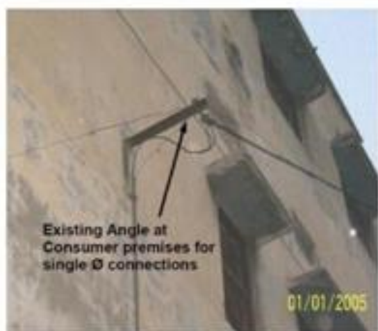
Fig. 1.26 Clamping arrangement on MS Angle
