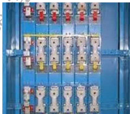
Fig. 1.29 Group Metering-Service Pillar
