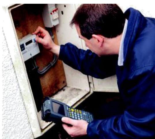
Fig. 1.9 Taking Reading from Electric Meter
