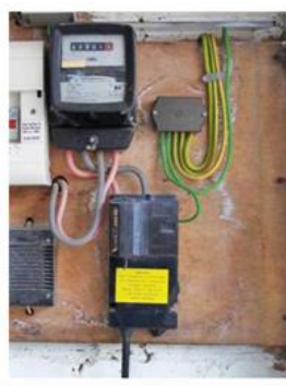
Fig. 1.46 Earthing in Electrical Meter
