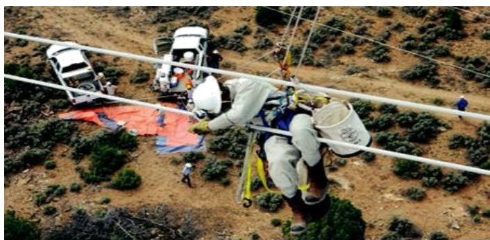
Fig. 4.13 Lineman Working with Rope
