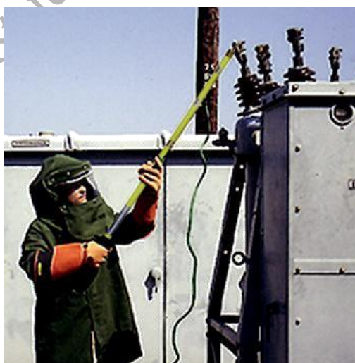
Fig. 4.8 Working with Discharge Rod
