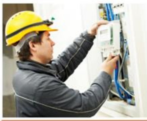
Fig. 1.37 Electrician Installing Energy Meter
