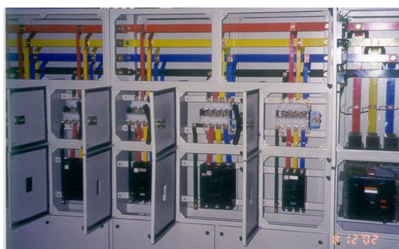
Fig 3.2 Another type of bus bar arrangement in Electrical panel
