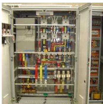
Fig 3.1 Bus Bar Arrangement in a Electrical panel
