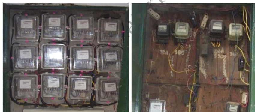
Fig. 1.24 Energy Meter Should Always be Installed in a Box of Utility Duly Sealed
