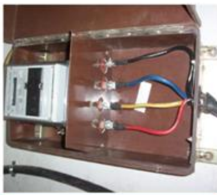
Fig. 1.34 LT CT Meter with Box
