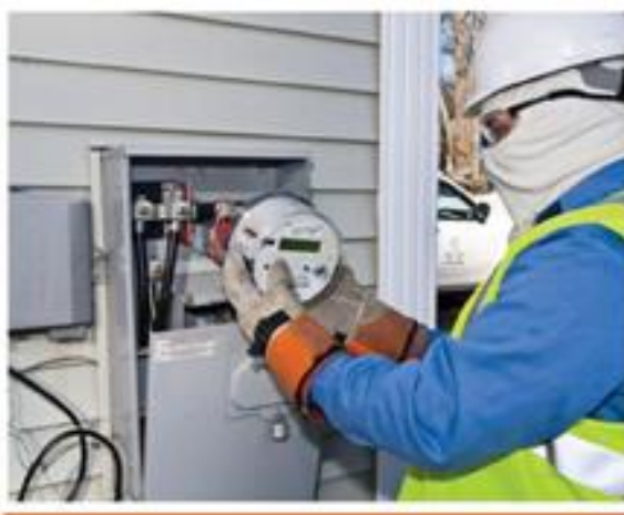
Fig. 1.38 Smart Meter Installation within Premises
